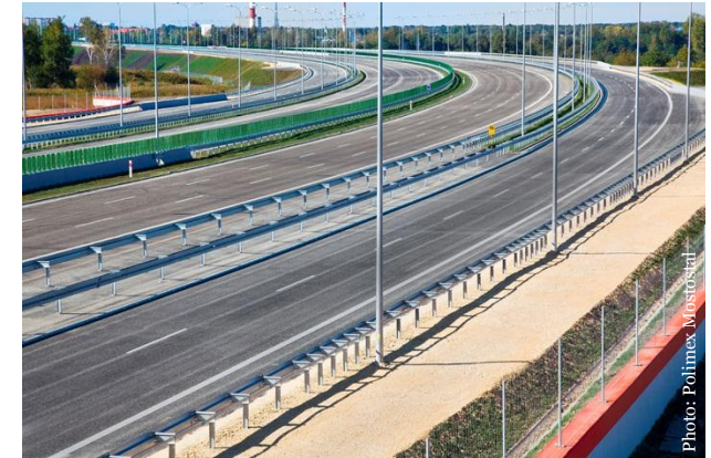
The newly finalised motorway A1, at the junction Sośnica – Maciejów in Poland, built by Polimex Mostostal, is one of East Capital's investments that benefits from the strong domestic demand in the country.
